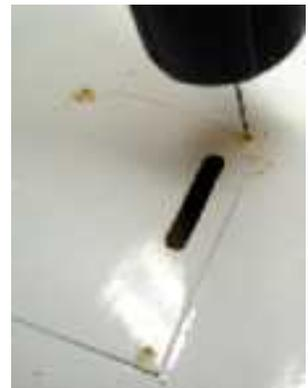
3) With the covers in place, drill a 1/16" (1.5mm) hole at each
